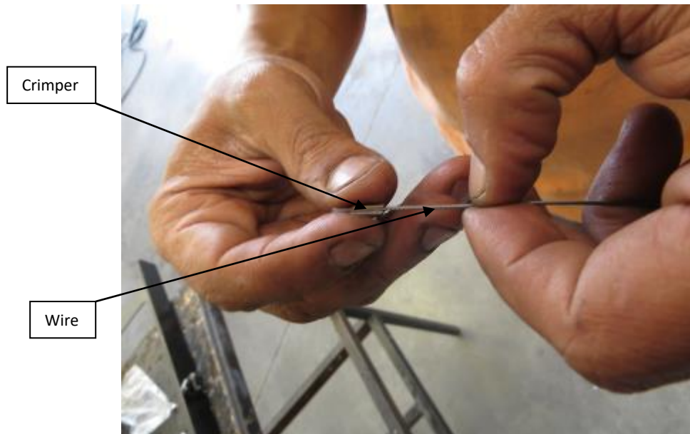
Figure 10: Inserting wire into 1 side of crimper
